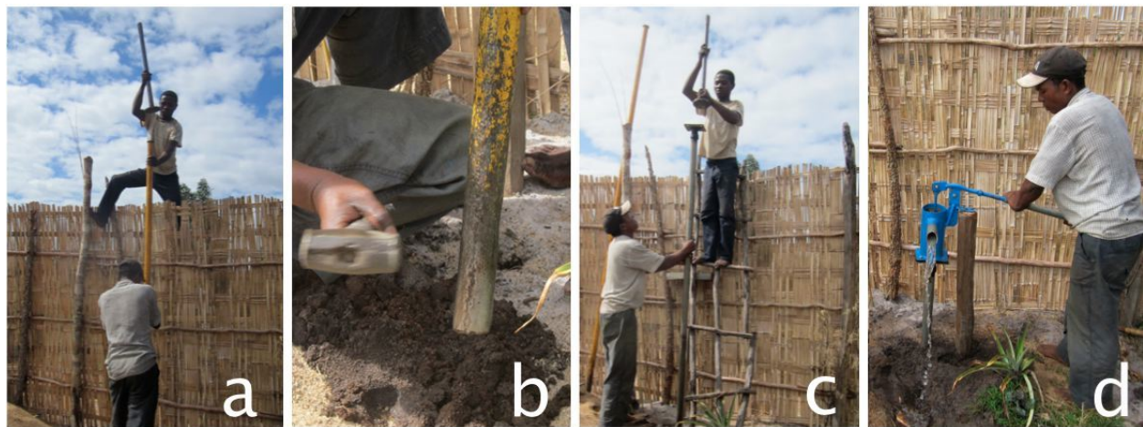
Figure 2. Typical installation of a Pompe Tany : a) percussion augering of soil; b) removed soil; c) percussion drilling of tube well/casing; d) finished pump.
